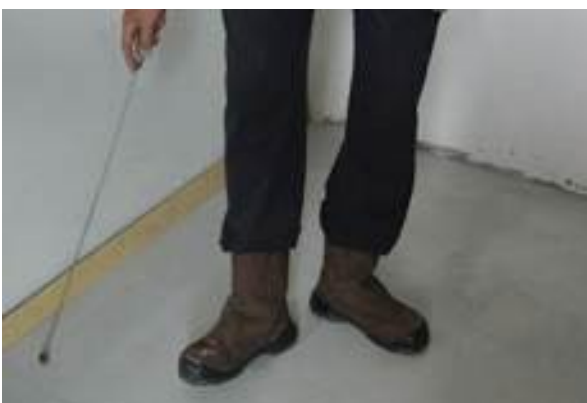
Checking substrate hollowness Figure 4.1.e
