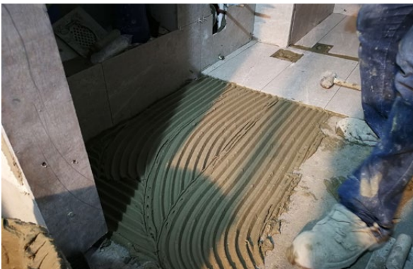
Adhesive fully trowelled Figure 5.2.c
