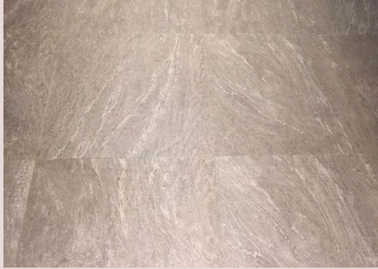
Good surface finishes Figure 5.5.e
