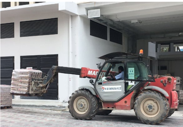
Sending materials for storage Figure 3.1.c
