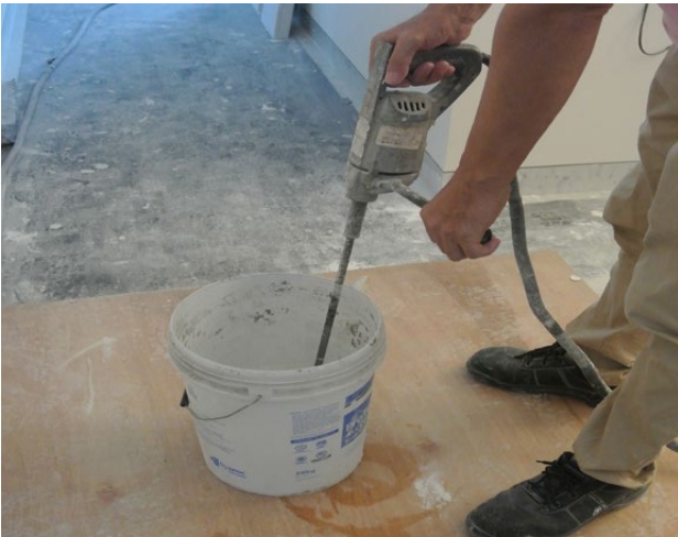
Mix with electric mixer Figure 5.1.c
