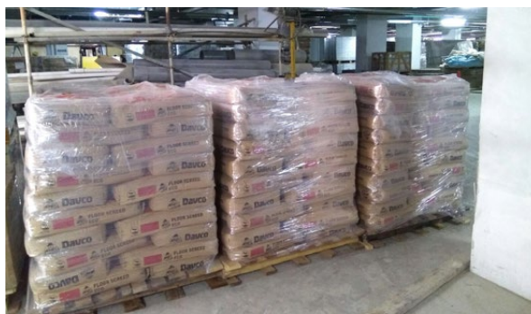
Proper storage of adhesives
