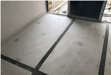
Laying of protection over completed floor tiles Figure 6.a
