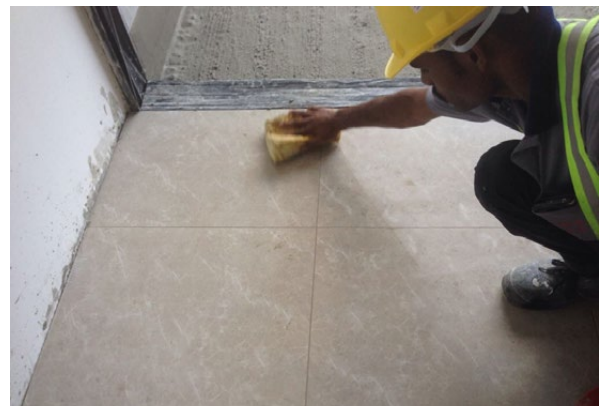
Removal of surplus grout Figure 5.3.d
