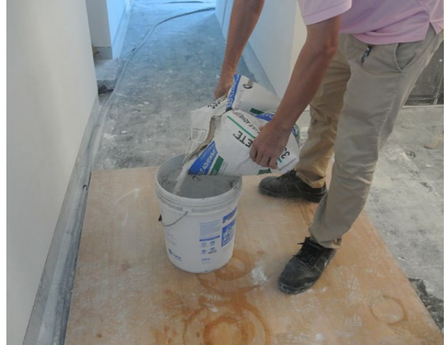
Adding powder into the container according to manufacturer's specs Figure 5.1.b
