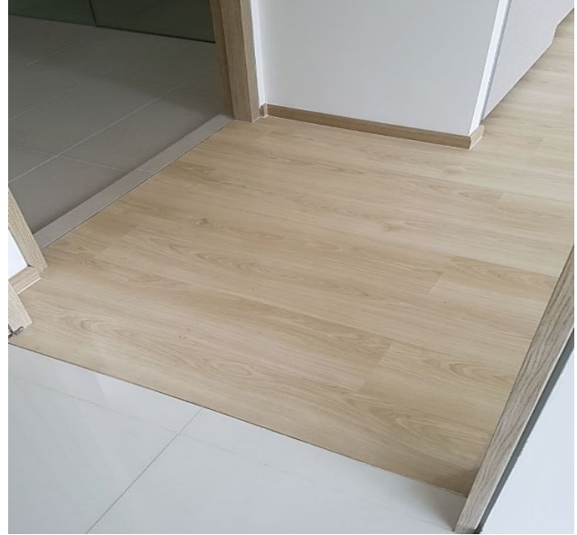
Neat joints at floor divider of completed unit Figure 2.3.1.b
