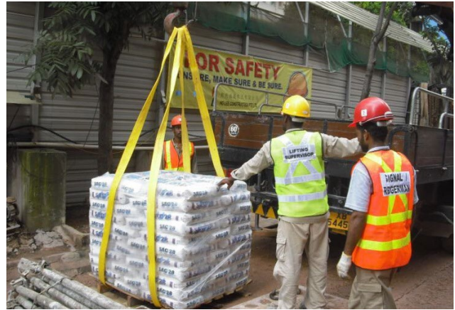
Offloading materials from lorry crane Figure 3.1.b
