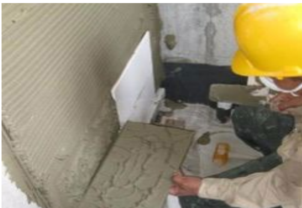
Installing tile on wall Figure 5.2.k
