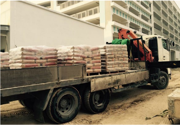
Transporting materials to site Figure 3.1.a
