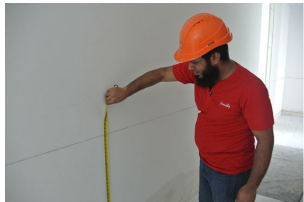
Checking level of surface Figure 4.1.d
