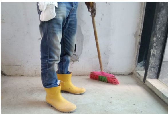
Cleaning surface with broom Figure 4.1.c
