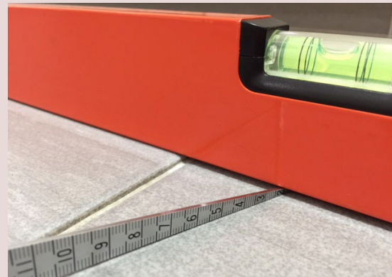
Lippage between tiles not more than 0.5mm Figure 5.5.l
