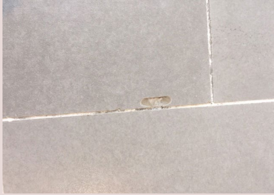
Chipping Figure 5.5.m
