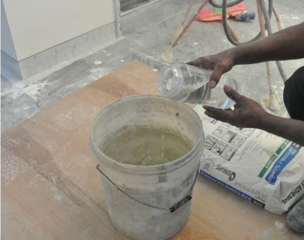
Amount of water or liquid latex added according to manufacturer's specs Figure 5.1.a
