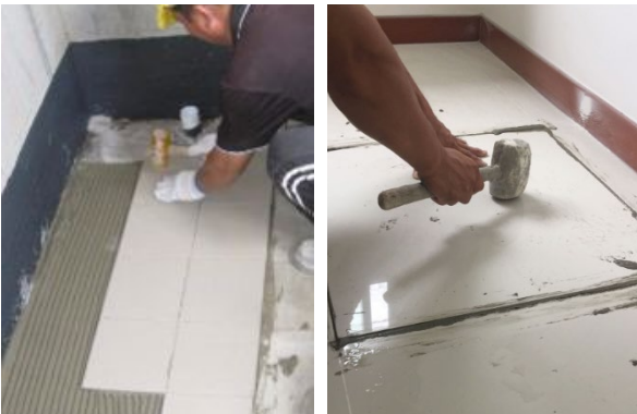
Using mallet to tap on tile for good coverage of tile adhesive between tile's back and floor substrate Figure 5.2.e
