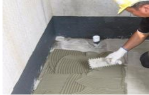
Trowelling adhesive with notched trowel Figure 5.2.b
