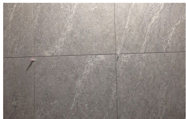
Plastic spacer for consistent joint Figure 5.2.h
