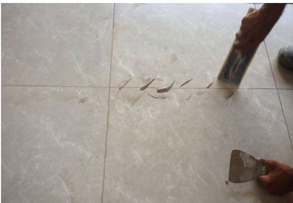
Filling of grout joints Figure 5.3.c
